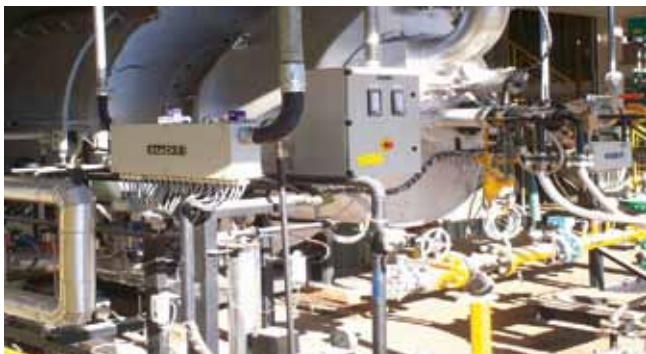
Versatile firing for molasses, natural gas, soybean oil and animal fat
